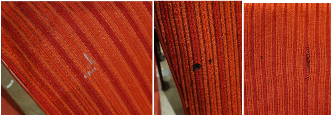
Figure 3: Detail of existing seating showing wear and material deterioration
