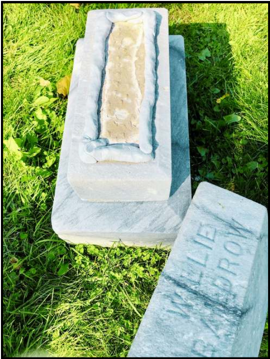
Above: Special fast-drying putty, which turns to cement, used to seal loose sections.
