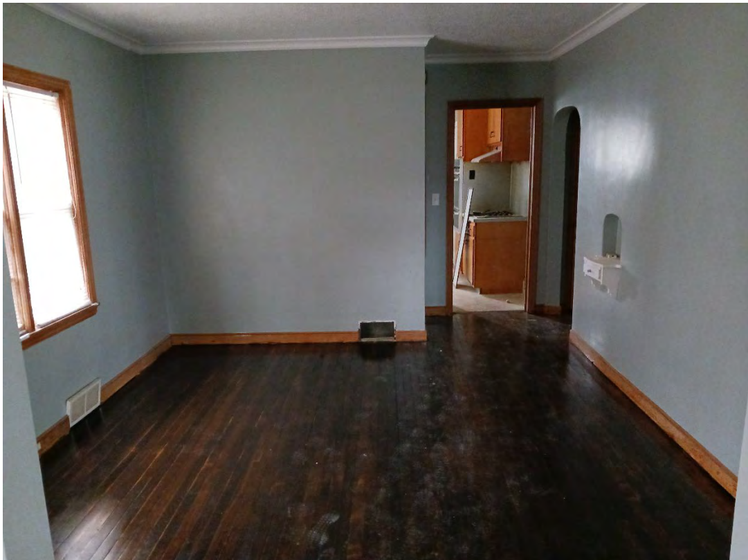
415 Cedar – First Floor Apartment 1 – Dining Room
