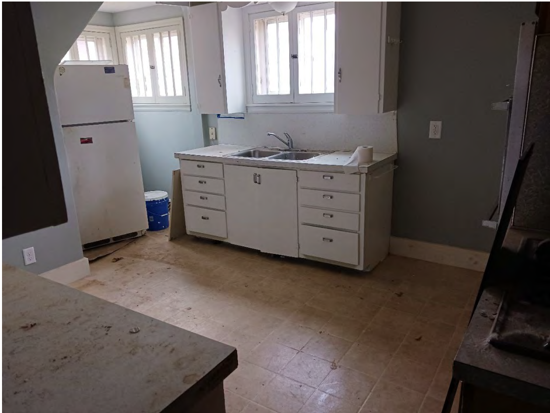
415 Cedar – First Floor Apartment 1 – Kitchen
