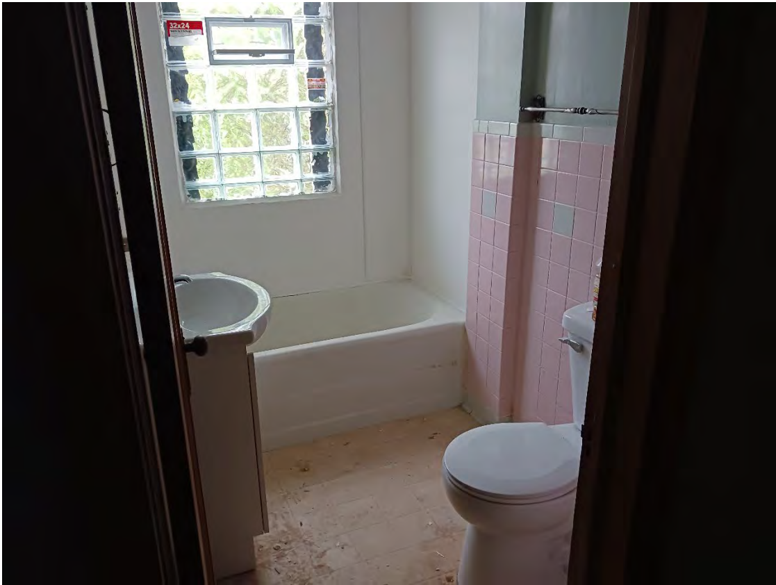
415 Cedar – First Floor Apartment 1 – Bathroom
